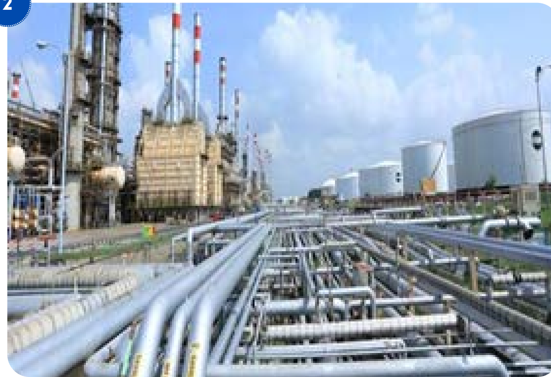
Material Procurement Of Shell Course, Shell Plate, Bottom Plate, Rolling Ladder, Line Foam, Floating Roof and Counter Weight in PT Pertamina RU IV Cilacap
