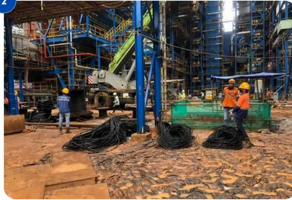
Electrical Work, Control & Instrument Work in Adaro Mining, East Kalimantan
