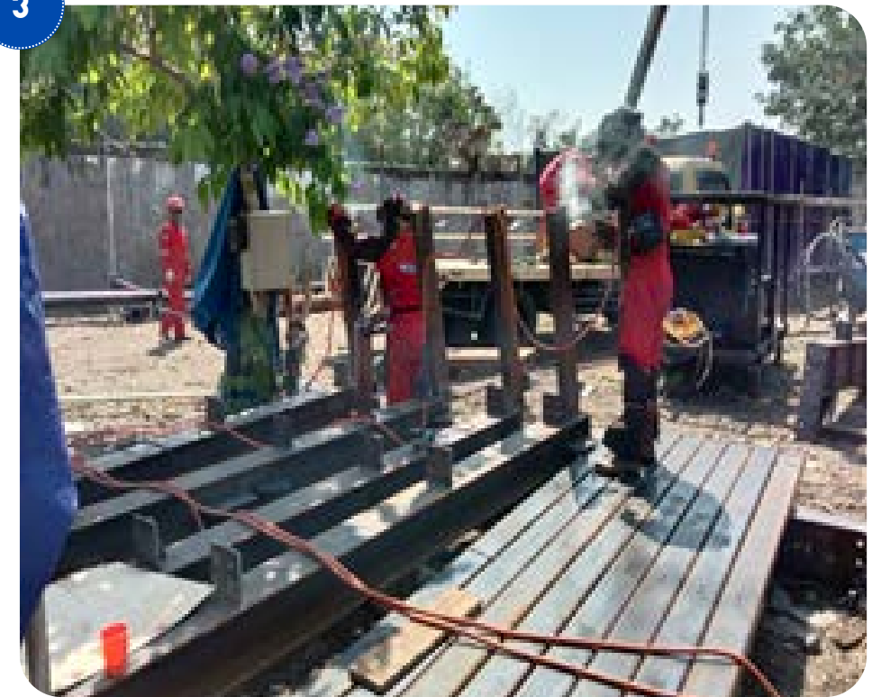
Gas Pipe Installation in Sequis Center and Jayanti Jakarta, PT Mayora
