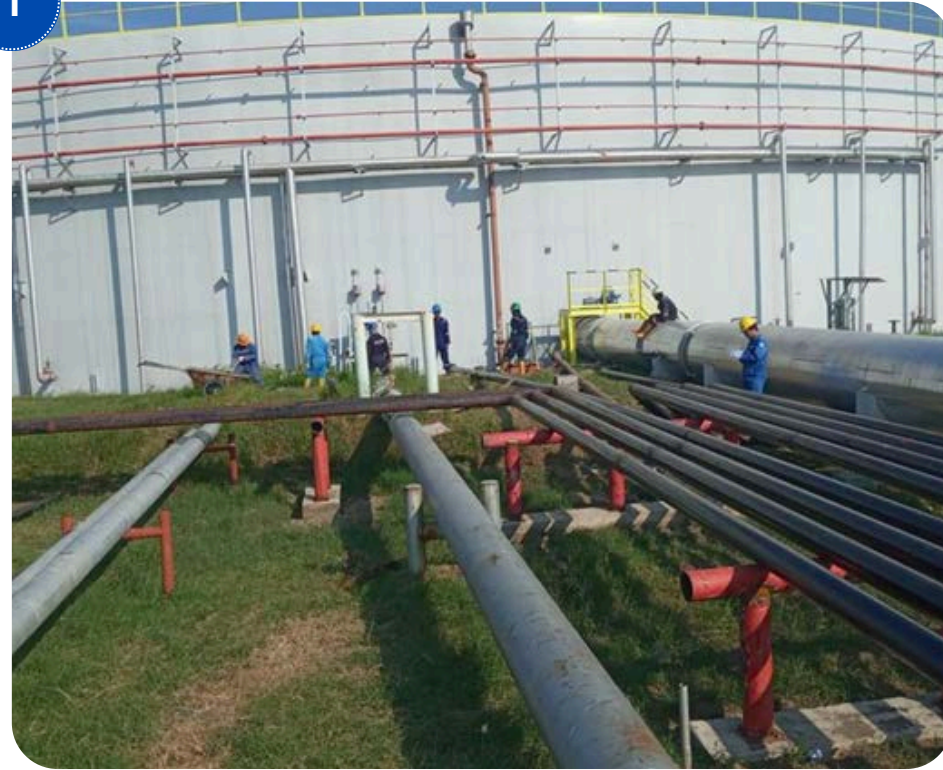
Improvement of Fire Protection System in Gathering Station Balongan Oil and Gas Transportation Field PT PERTAMINA EP Zona 7
