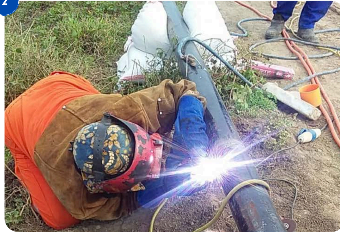
Maintenance of Pipeline Facilities in Jatibarang Field, PT Pertamina EP Asset 3
